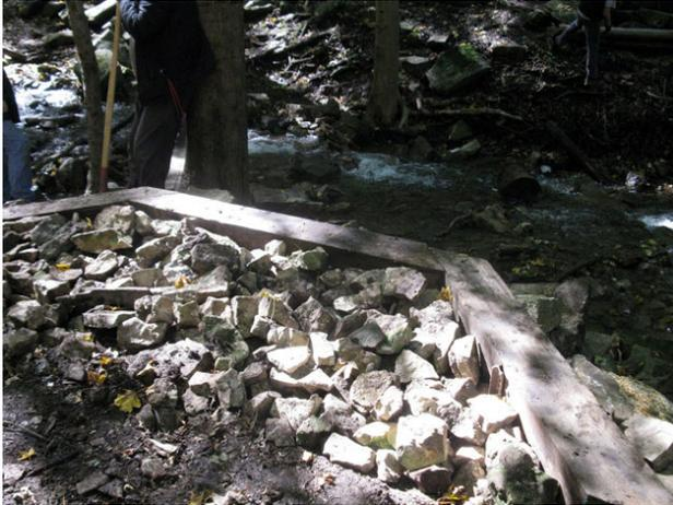
The footings at each end of the bridge were reinforced. Wooded beams, 8"x8" were used plus logs, placed in a configuration to contain the existing supportive rock. Additional rock was added. The banks of the streambed were also reinforced to reduce the possibility of erosion. This part of the reconstruction was a two-day project in itself. Tons of rock were moved manually by our volunteers on each of the two days.
